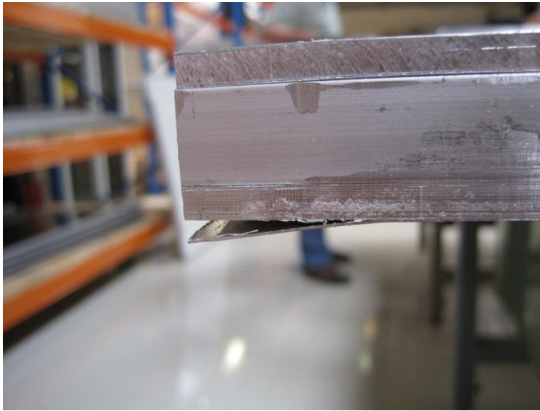
Delamination due to insufficient bonding as a result of lack of glue.
