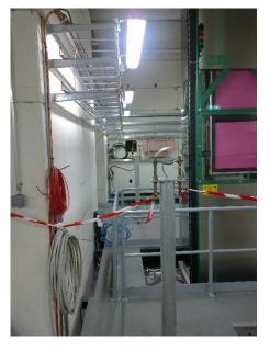
If the cable trays are put higher up or flush against the wall then the translation distance goes from 30 cm to 1.6 m
