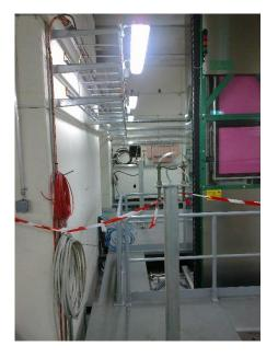
If the cable trays are put higher up or flush against the wall then the horizontal translation distance goes from 30cm to 1.6m.
