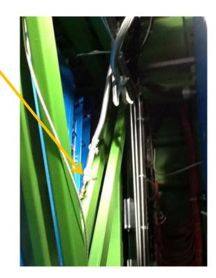
1 supply and 1 return pipe (per side) arrive only to the X2 balcony level on YE1 (i.e. the part from X2 to X3 and the cable chain is missing)
