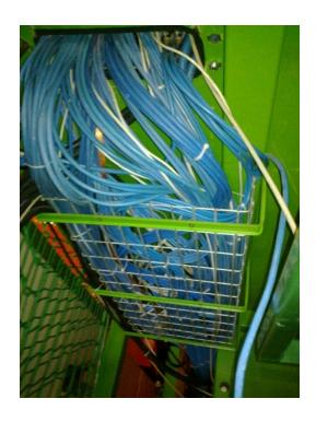
Cables on the front of the rack from Trigger LV will have to be moved to the side of the floor access
