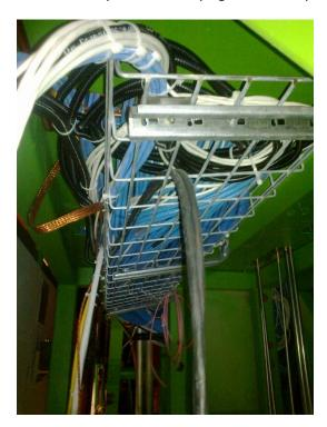
The first sector fitted with dummy patch panels for the cabling of the Signal and finalising of the HV cables.
