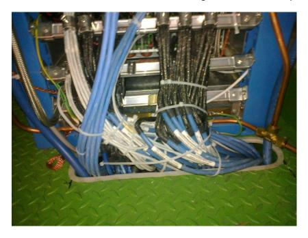
Here we need a new cable tray just under this one BUT starting from the back of the rack. This will allow the big red CSC cables to be cabled correctly. See  $2^{nd}$  photo.
