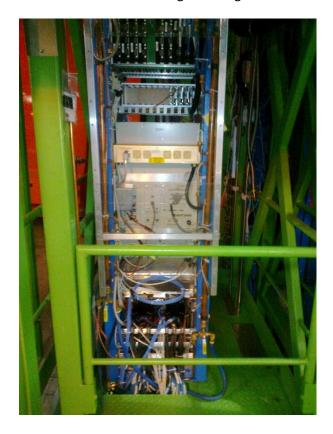
This cable tray needs modifying as it is collapsing. A new one in addition is required.
