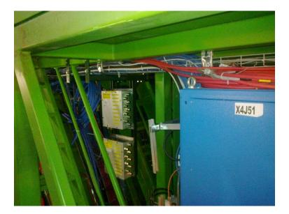
In addition the black boxes mounted at the rear of the rack block access to the LBB back plane.
