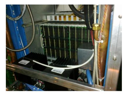
We will need a cable tray 200mm wide installed under the rack floor under the present one.
