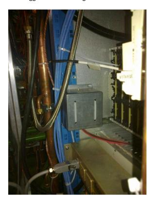
The cabling in this rack must be cleared up, it seems to primarily concern the cables for the trigger.
