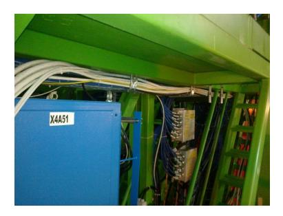
The cabling at the top of the rack is poorly done and now will limit access to the additional RE4 cabling tray. Behind the panel shown below the black boxes have to go.
